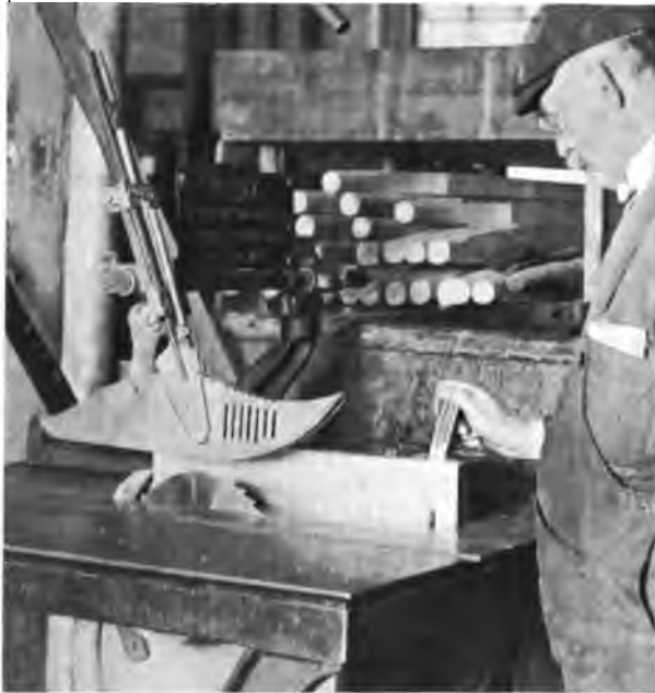
Fig. 1. Guarded Circular Saw.*
